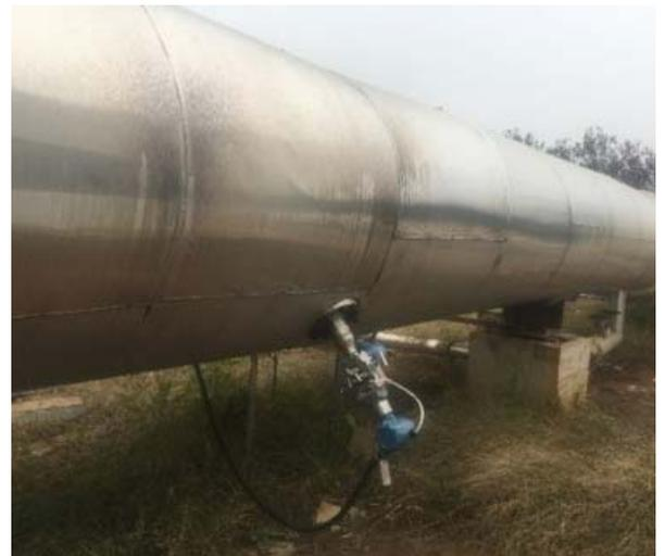
measurement. The instrument measures differential pressure, static pressure, and process temperature in a single device while dynamically calculating mass flow 22 times per second within the transmitter.
