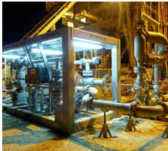
Micro Motion Coriolis High Capacity sensor installed after the choke
