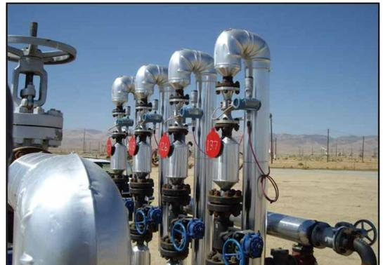
A ball trap connected to a turbine meter was used to measure oil flow from one of seven producing oil wells on any given header. A Rosemount 8800 MultiVariable vortex meter with a WirelessHART THUM now provides a low-maintenance option that gives continuous, one-minute updates for each individual well.
