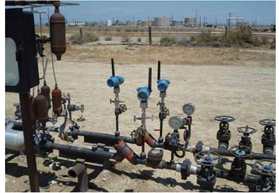
3051S WirelessHART pressure transmitters on a dual injection stream well.
