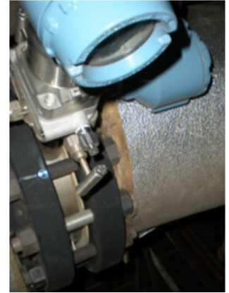
Rosemount Compact Annubar Flow Meter installed between two raised-face flanges
