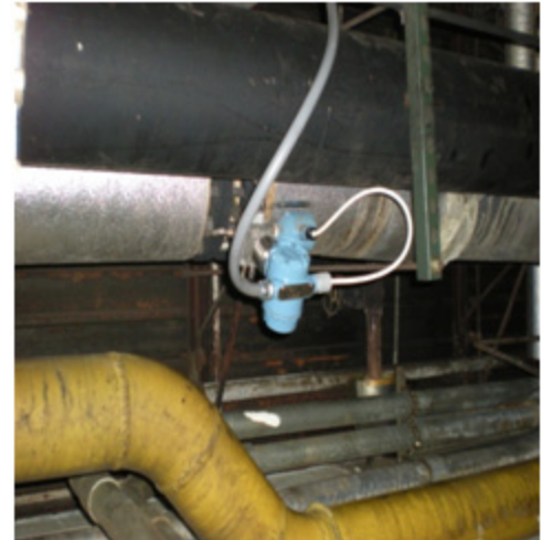
Rosemount Compact Annubar Flow Meter installation
